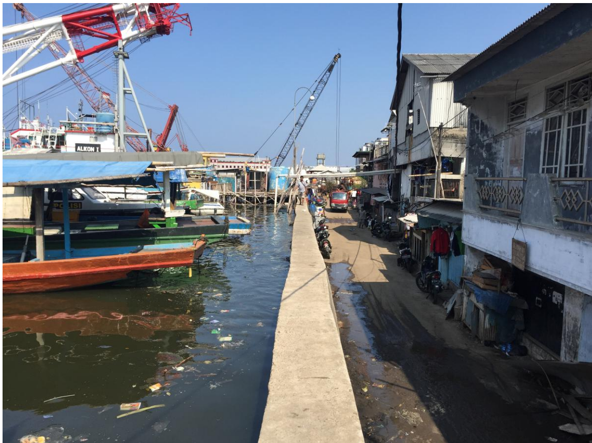
Figure 1. The current sea wall at Pluit in North Jakarta, 2015 (source: Author).
