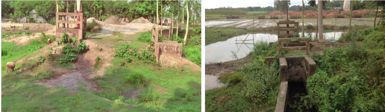
Figure 3. Images of a broken-down main regulator sluice gate (left) and soil accumulation inside the inlet (right).
