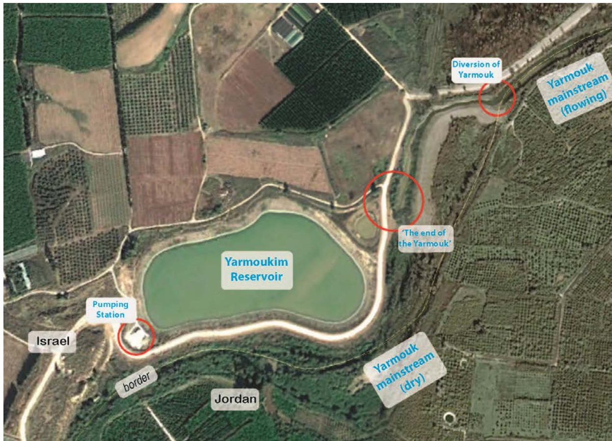
Figure 5. The 'end of the Yarmouk'. Top: the Yarmoukim Reservoir showing the diversion and termination of the Yarmouk. Bottom: the reservoir and the motors of the four pumps.
