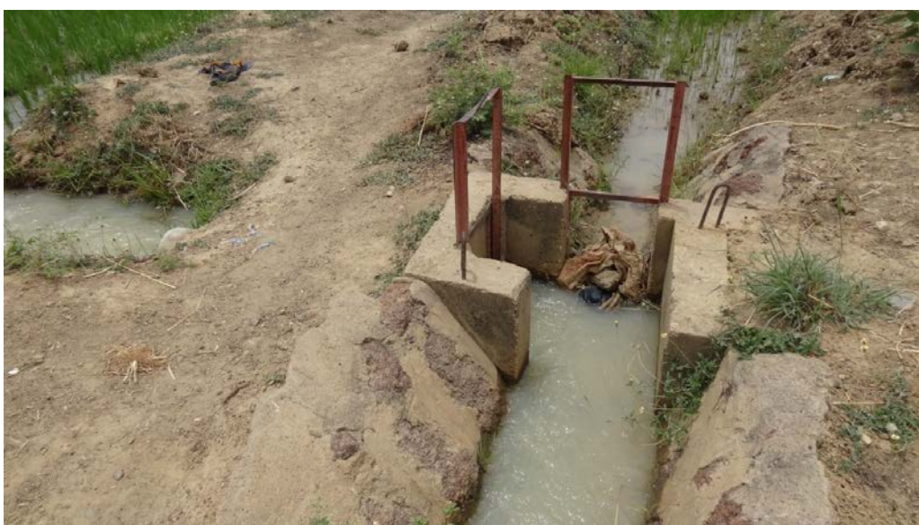
Figure 2. Waterways clogged with stones, grass, and worn clothes, which slow down the flow.
