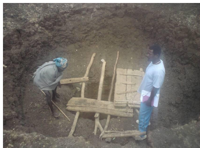
Figure 5. Construction of a V-shaped well.
