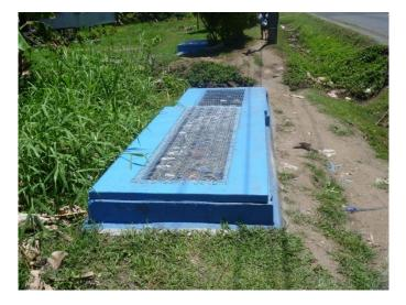
Figure S2. New connection to water mains in Fiji Settlement 2. Source: authors.
