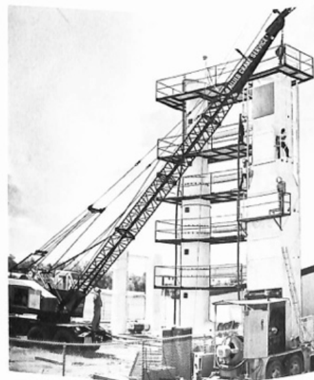
FIGURE 111.—Peñasco pilot plant evaporator-condenser unit (under construction at Tucson).
