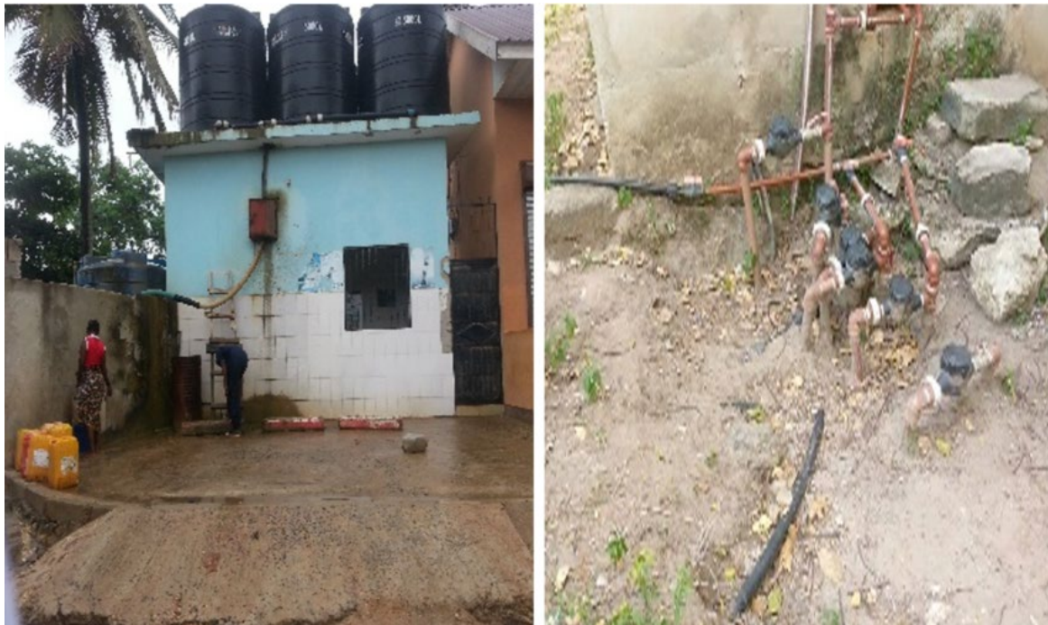
Figure 2. Privately mechanised borehole networked water system.
