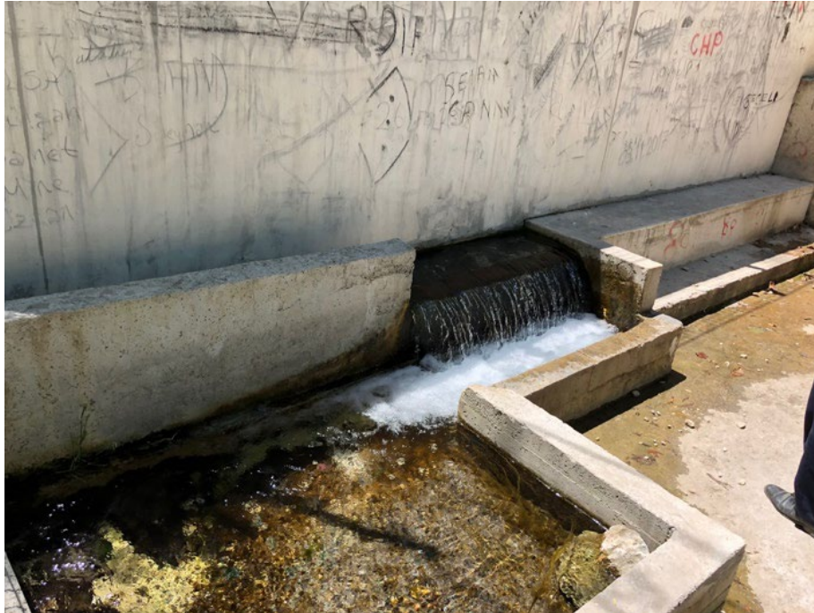
Figure 3. The concrete hut enclosing the water source.
