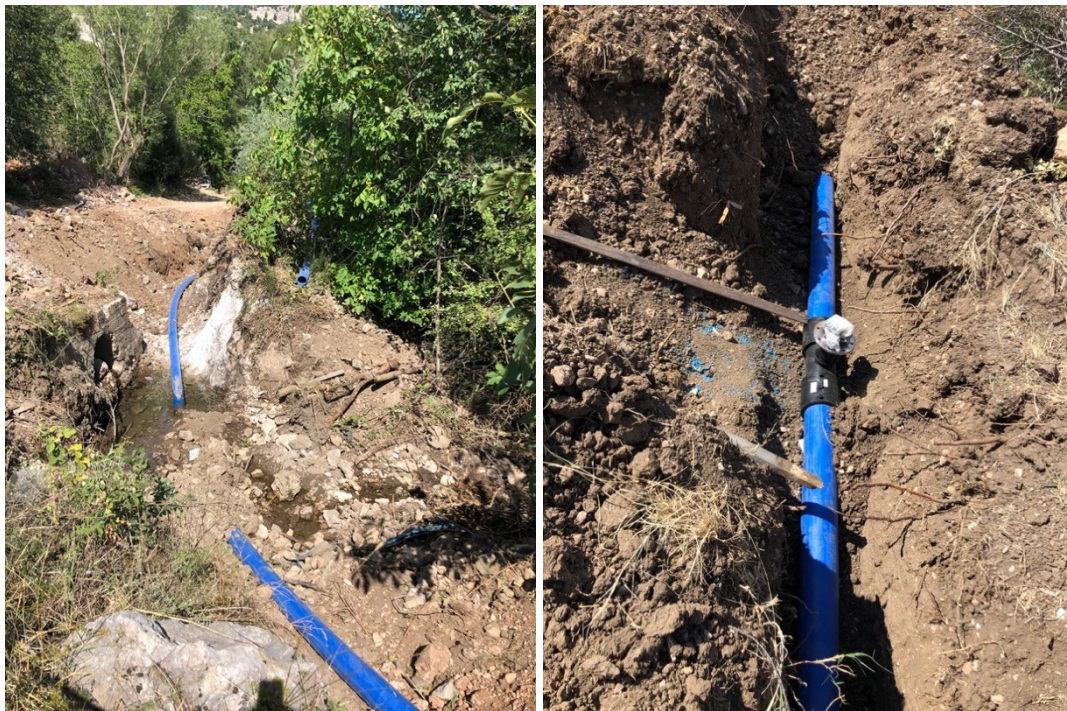
Figure 6. The drip irrigation infrastructure being built by the Ağlasun municipal government.
