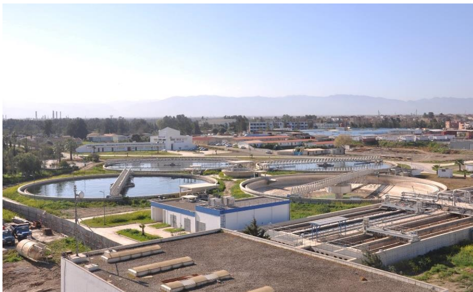
Figure 5. Wastewater Treatment Plant in Baraki, Algiers (2019).
