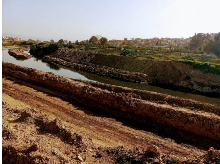
Figure 4. Oued El Harrach during depollution works.
