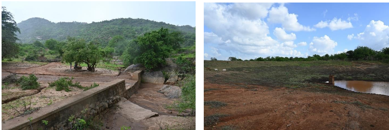
Figure 7. Sand dam (left) and water pan (right) constructed by a local NGO (Sahelian Solutions Foundation, or SASOL) and funded by international donors
