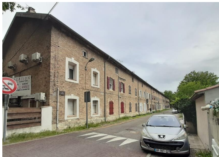
Figure 13. Industrial housing associated with salt production in Salin-de-Giraud
