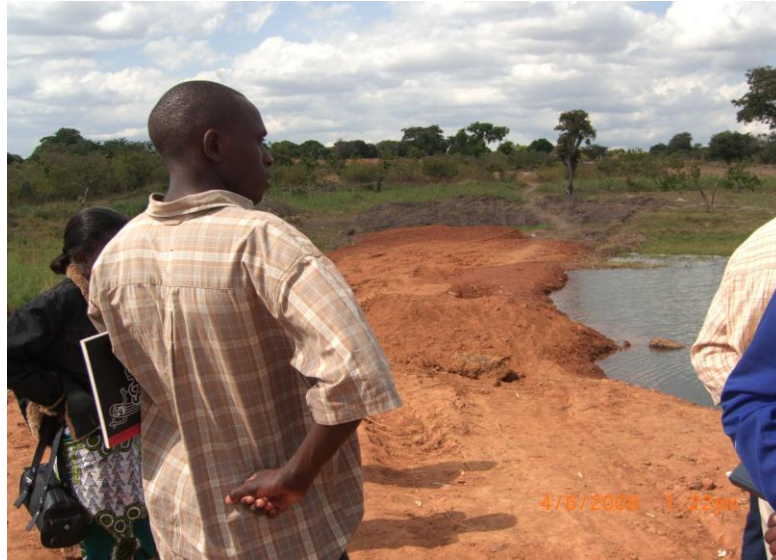
Figure 3. The uncompleted Chidika dam in Euthini, Mzimba.
