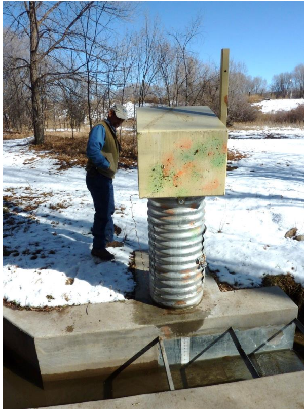
Figure 3. A Las Vegas (New Mexico) irrigator inspects a water gauge placed on a too-narrow flume, itself imposed on an older earthen acequia.
