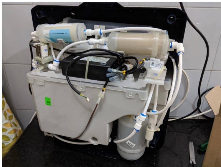
Figure 3. A reverse osmosis (RO) water purifier.
